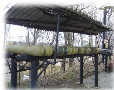
*Figure 7: Storage of Chlorine at WTP*
