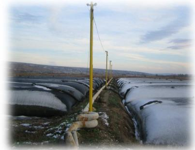
**Figure 12: Geotubes at WWTP**
