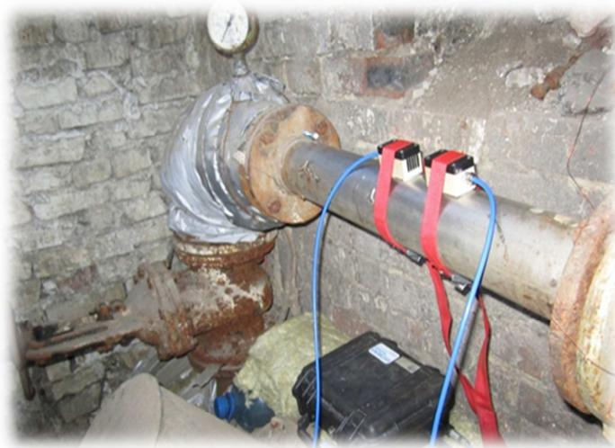
**Figure 26: Portable ultrasonic flowmeter installed in S.A. BUCURIA**
