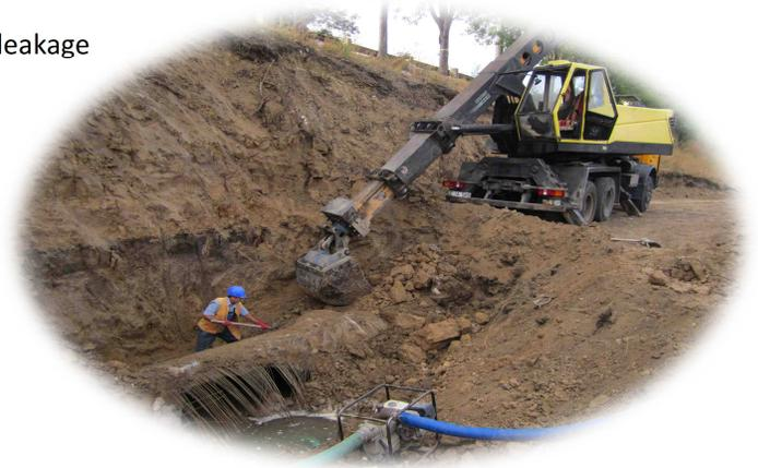
**Figure 9: Burst on a ND1200 cement pipe threatening the road**
